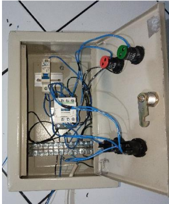
Gambar 8. Instalasi Panel Kontrol
