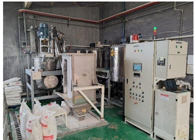
Gbr. 1 Mesin Glue Kitchen PT Surindo Teguh Gemilang 1
