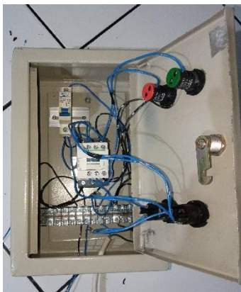
Gambar 8. Instalasi Panel Kontrol
